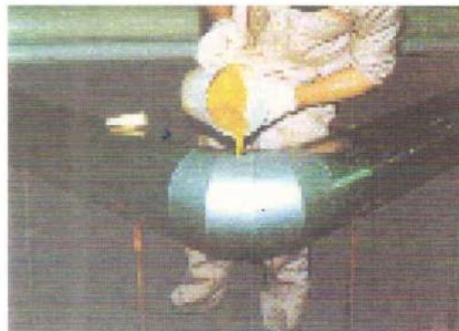
Pour Chemicals through opening
