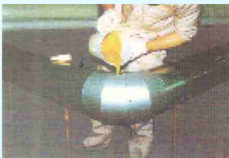
Pour Chemicals through opening
