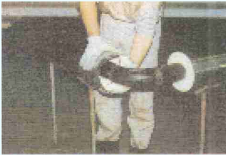
Place sleeve in position
